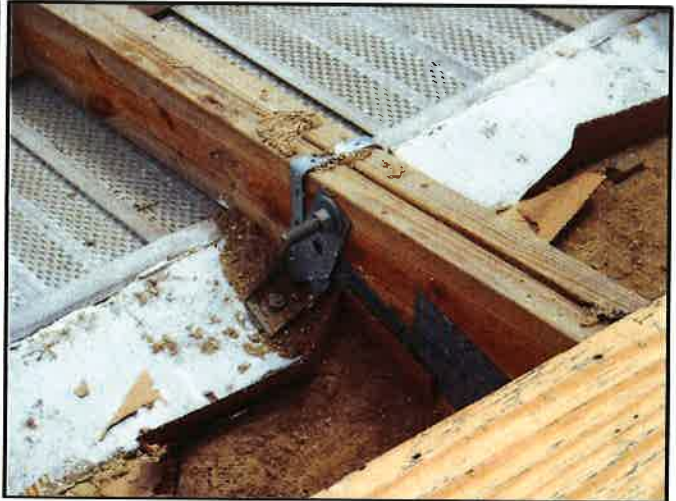
Double Truss Connection
