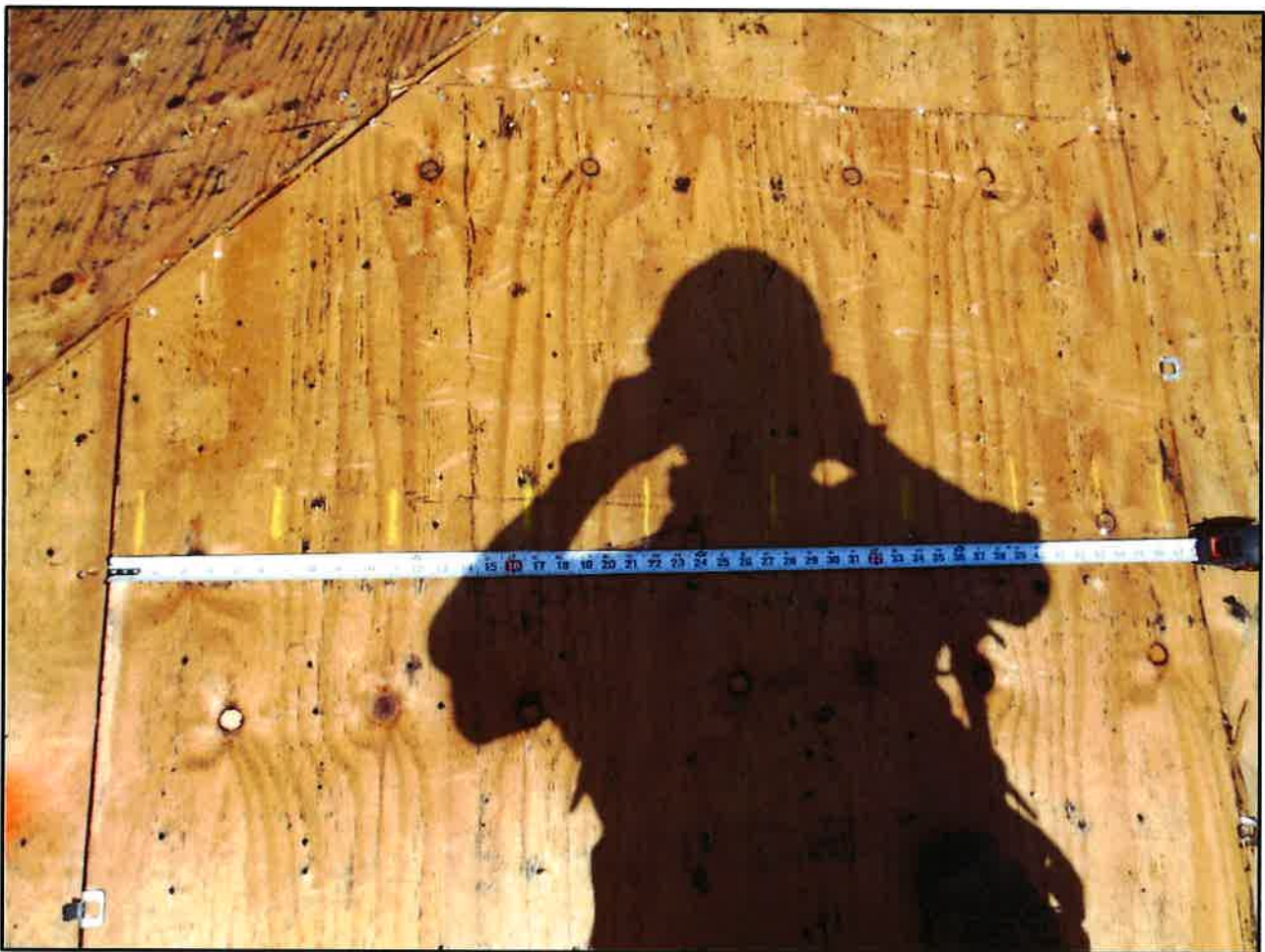
Plywood Nailing
