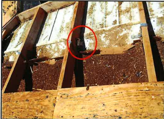
Truss to Wall Reinforcement
