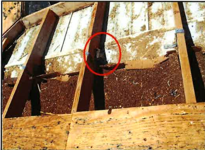
Truss to Wall Reinforcement
