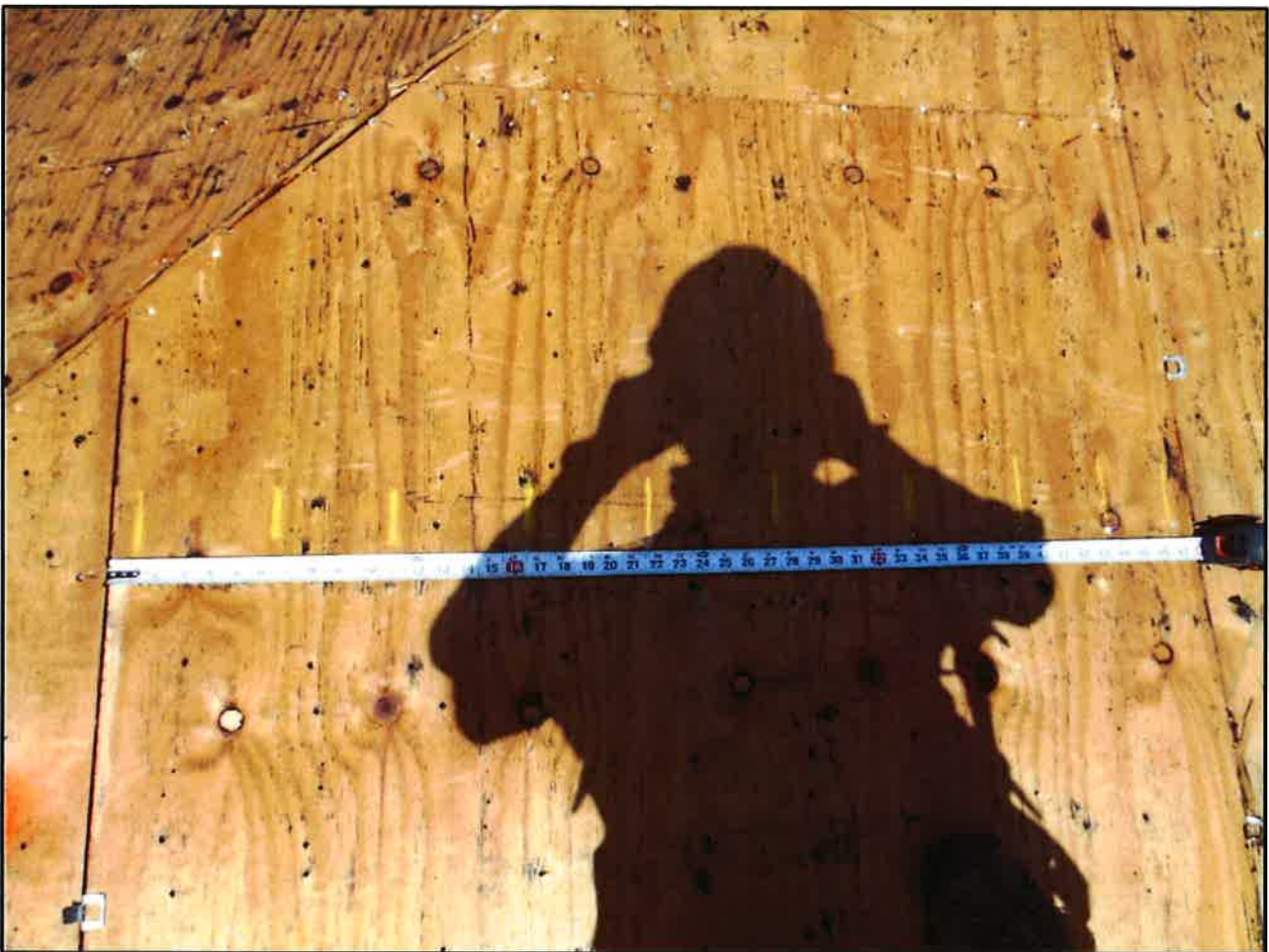
Plywood Nailing
