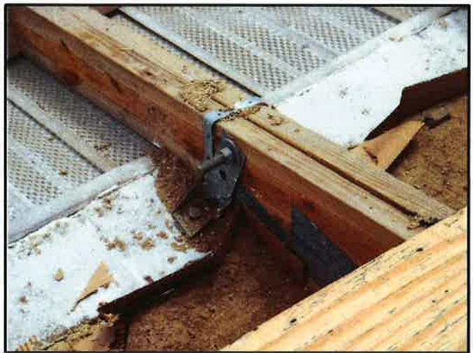
Double Truss Connection
