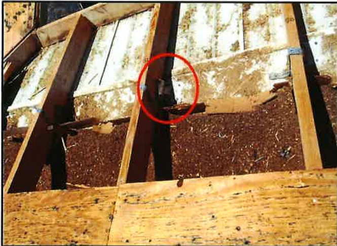
Truss to Wall Reinforcement
