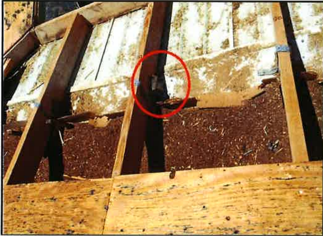
Truss to Wall Reinforcement
