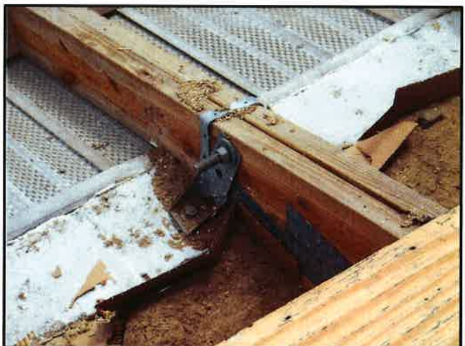
Double Truss Connection
