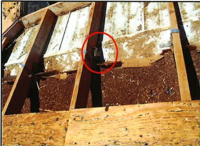
Truss to Wall Reinforcement
