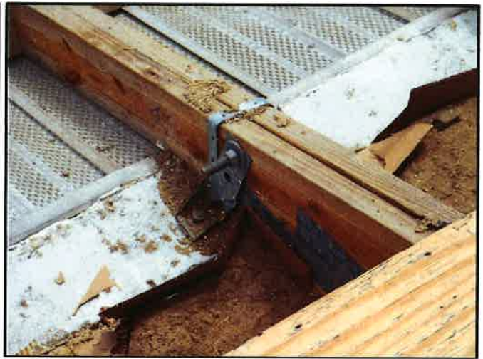
Double Truss Connection
