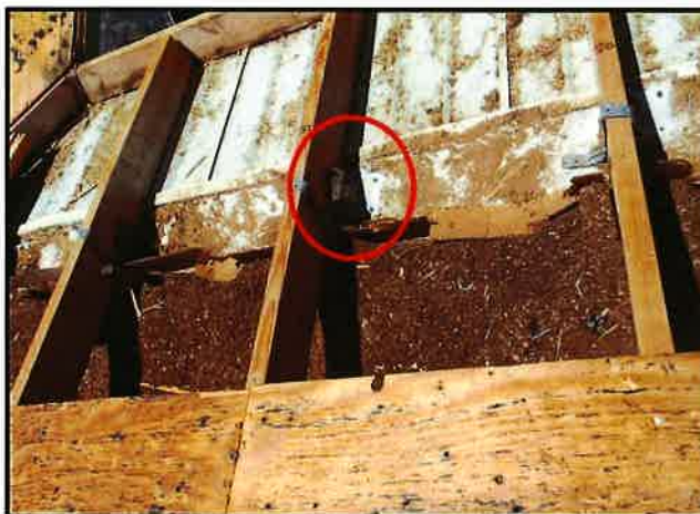
Truss to Wall Reinforcement
