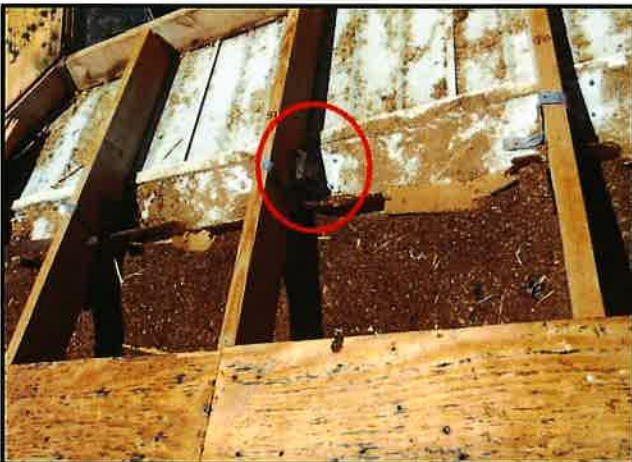
Truss to Wall Reinforcement
