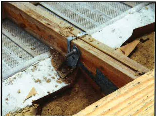
Double Truss Connection
