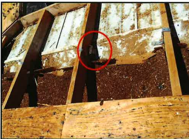
Truss to Wall Reinforcement
