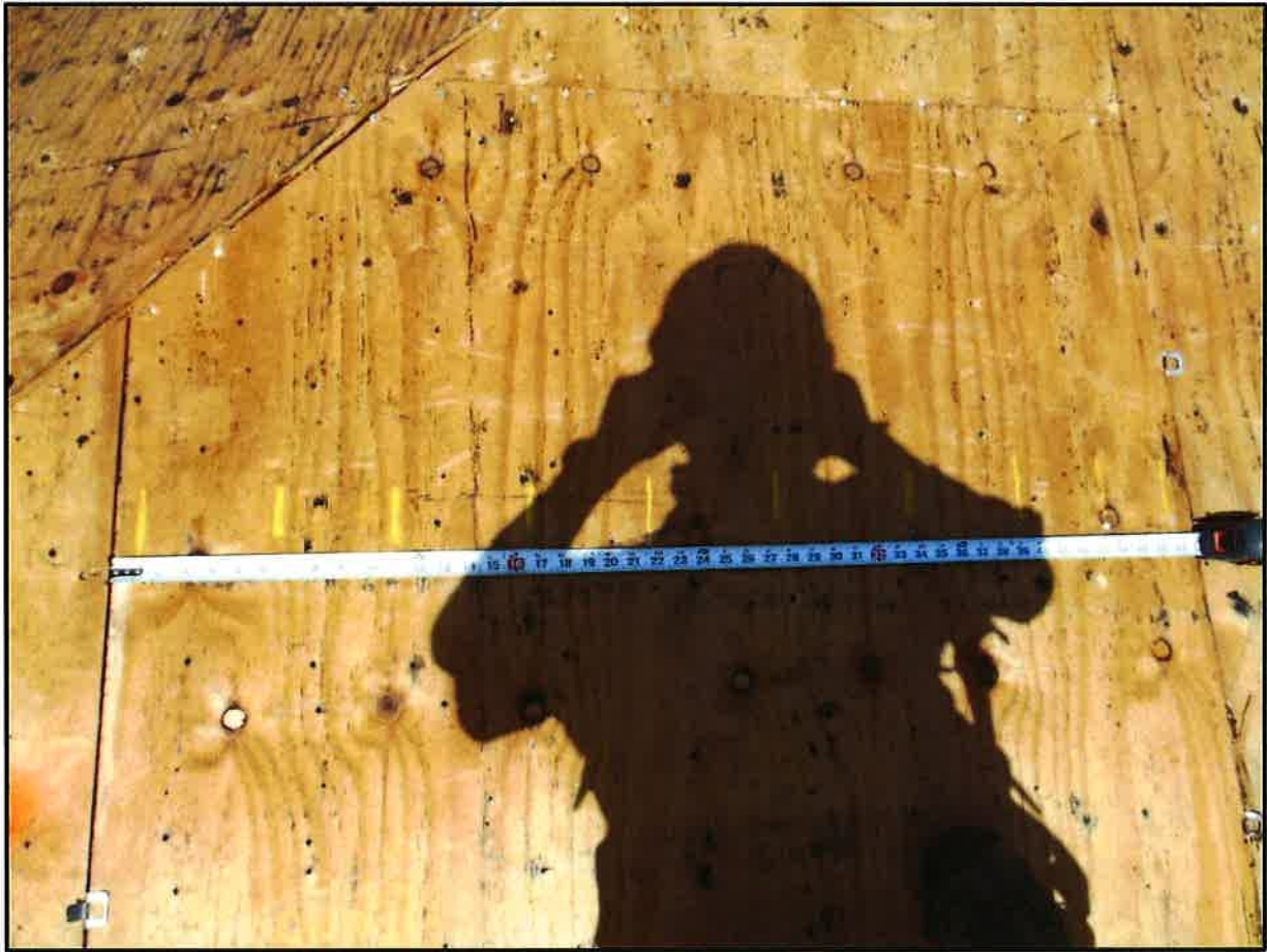
Plywood Nailing
