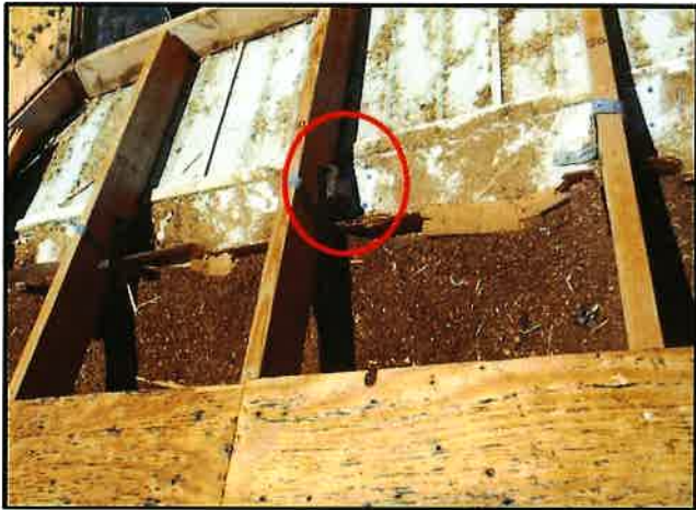
Truss to Wall Reinforcement
