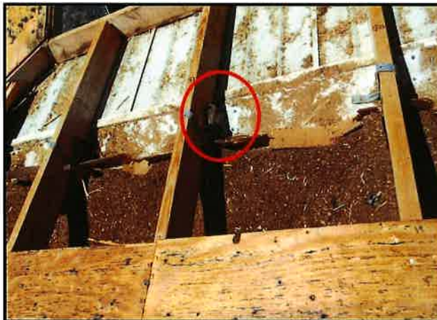
Truss to Wall Reinforcement
