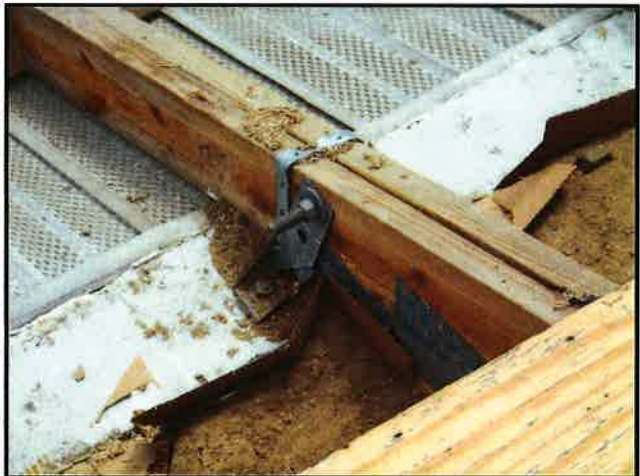
Double Truss Connection
