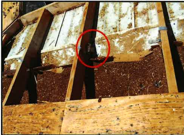
Truss to Wall Reinforcement
