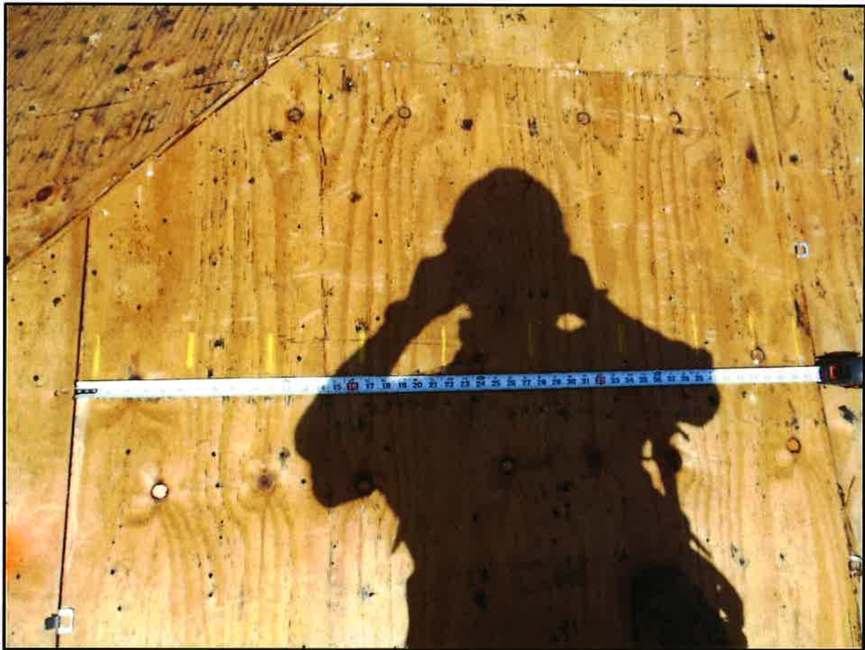
Plywood Nailing
