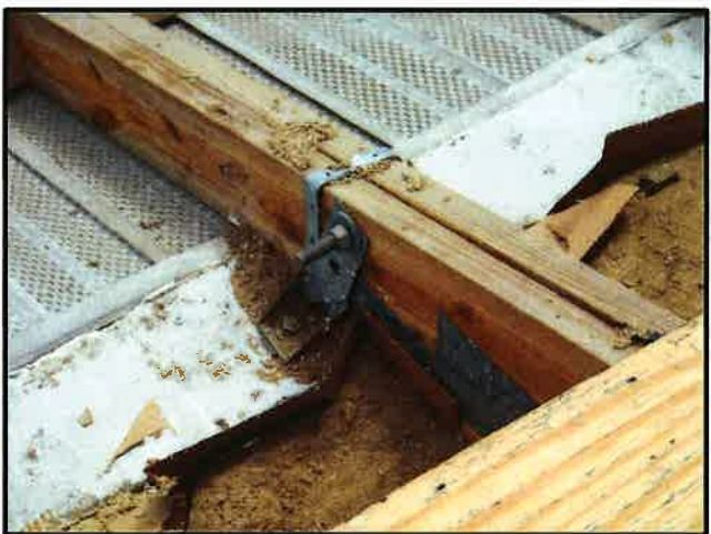
Double Truss Connection
