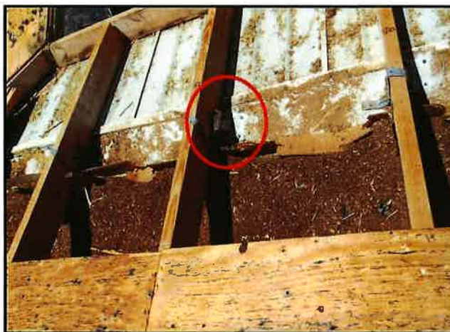
Truss to Wall Reinforcement
