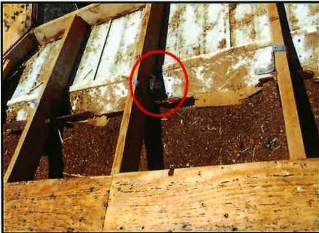
Truss to Wall Reinforcement
