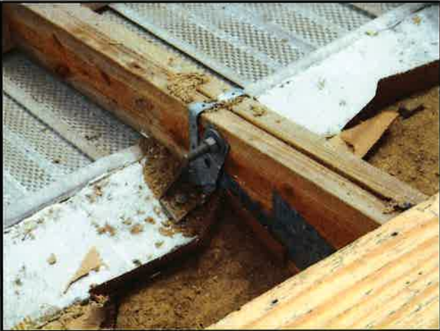
Double Truss Connection
