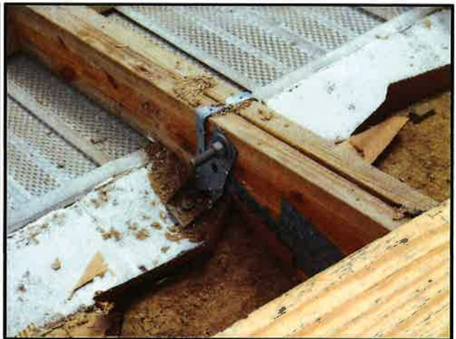
Double Truss Connection
