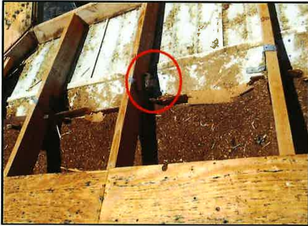
Truss to Wall Reinforcement
