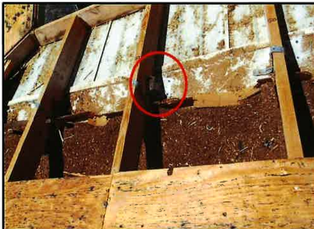
Truss to Wall Reinforcement
