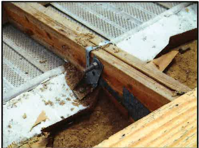
Double Truss Connection
