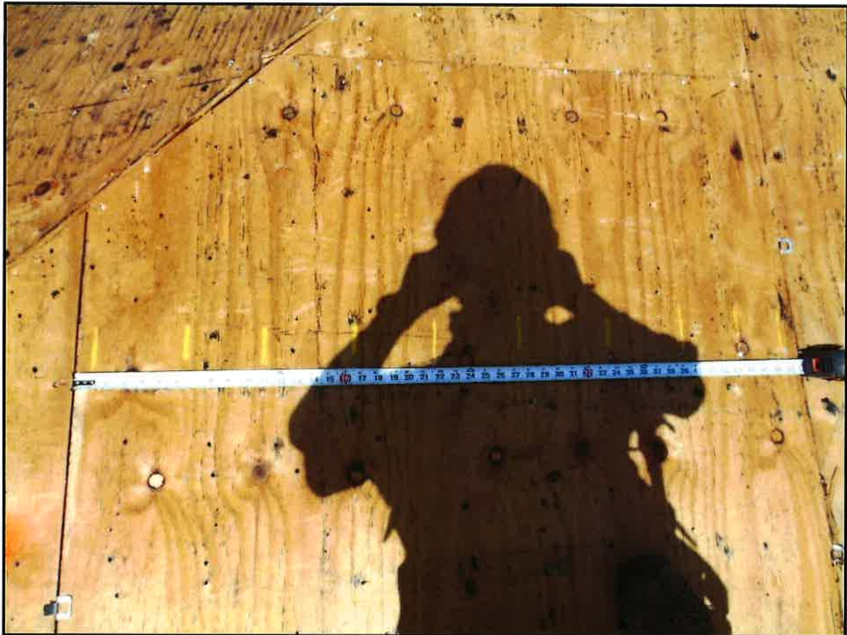
Plywood Nailing
