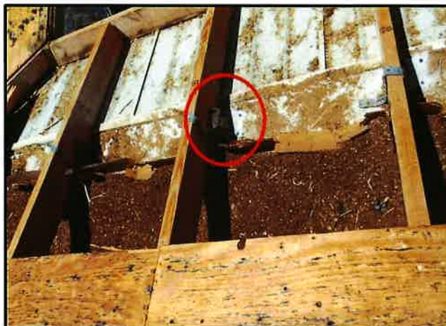
Truss to Wall Reinforcement
