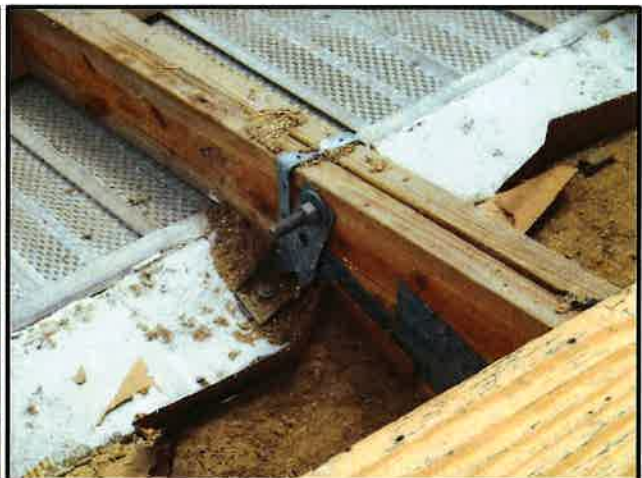
Double Truss Connection
