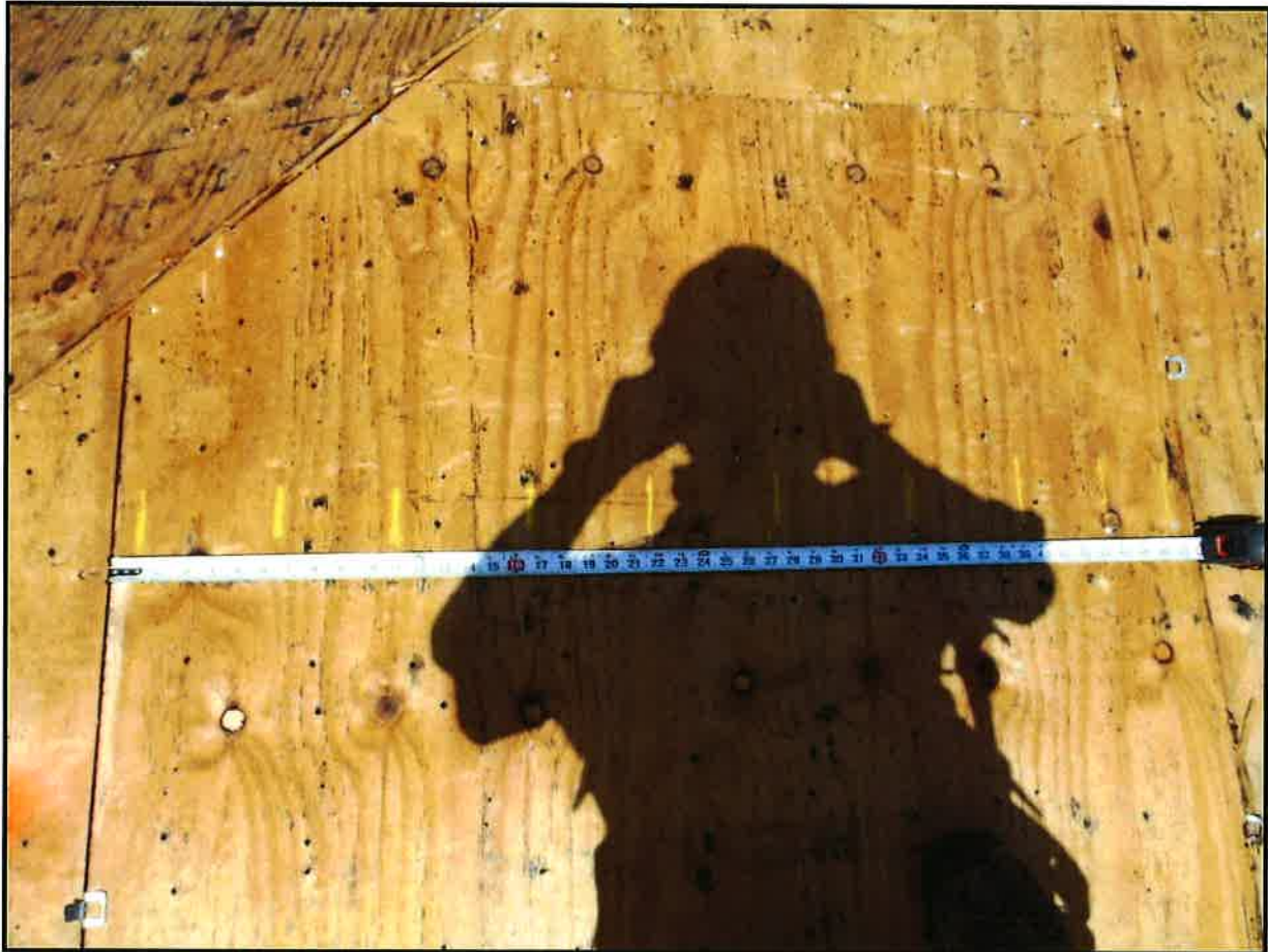
Plywood Nailing
