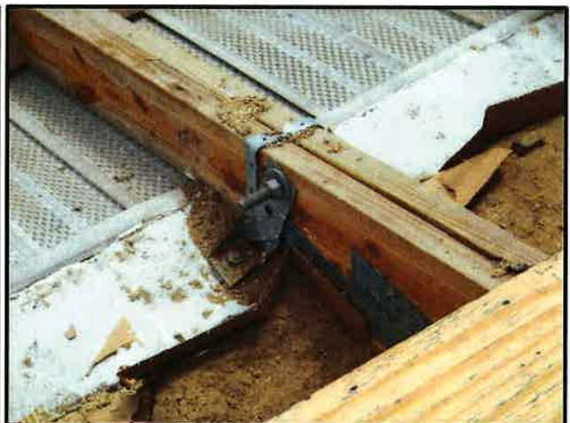
Double Truss Connection
