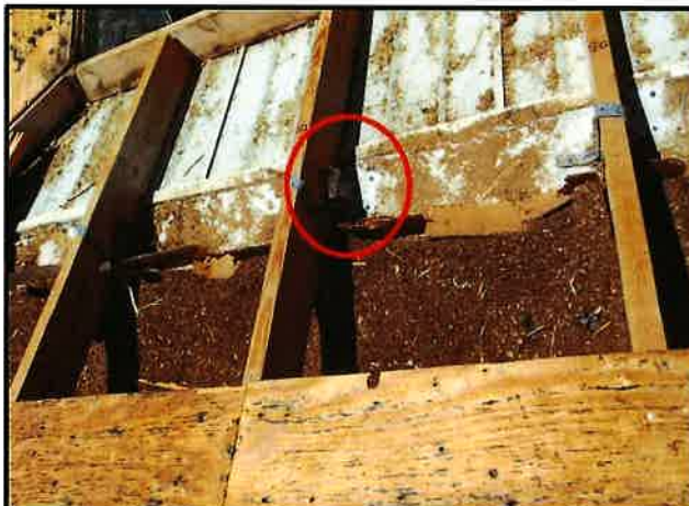
Truss to Wall Reinforcement
