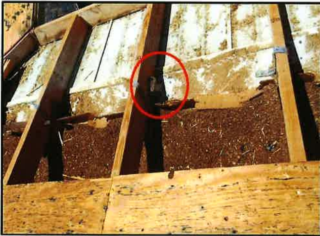
Truss to Wall Reinforcement
