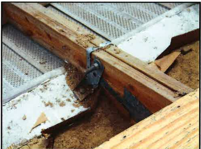
Double Truss Connection
