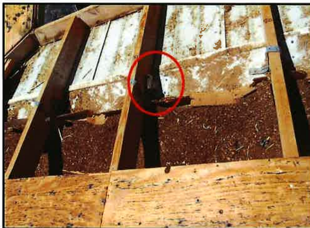
Truss to Wall Reinforcement
