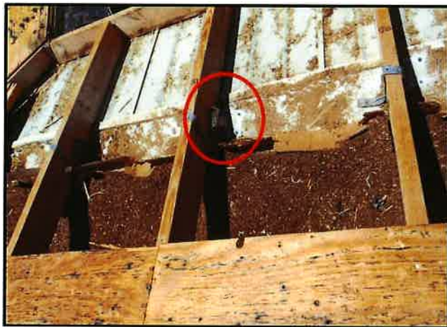
Truss to Wall Reinforcement
