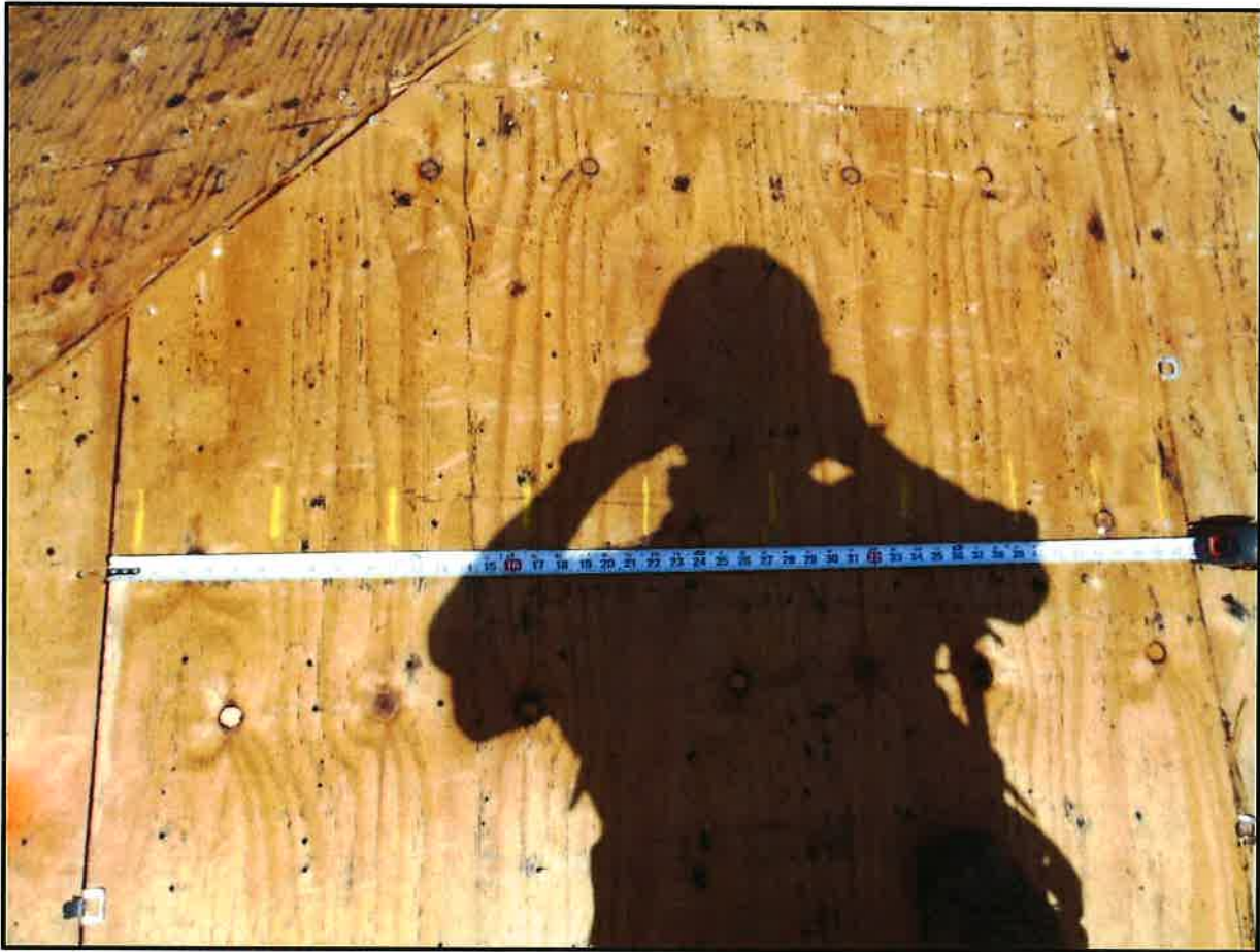
Plywood Nailing
