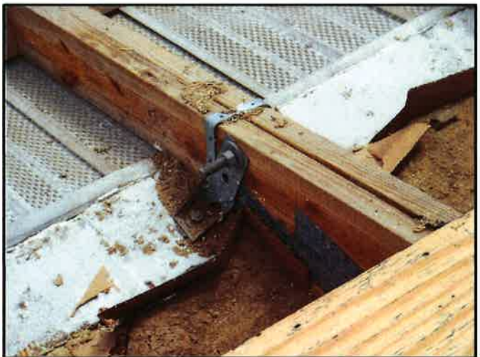
Double Truss Connection
