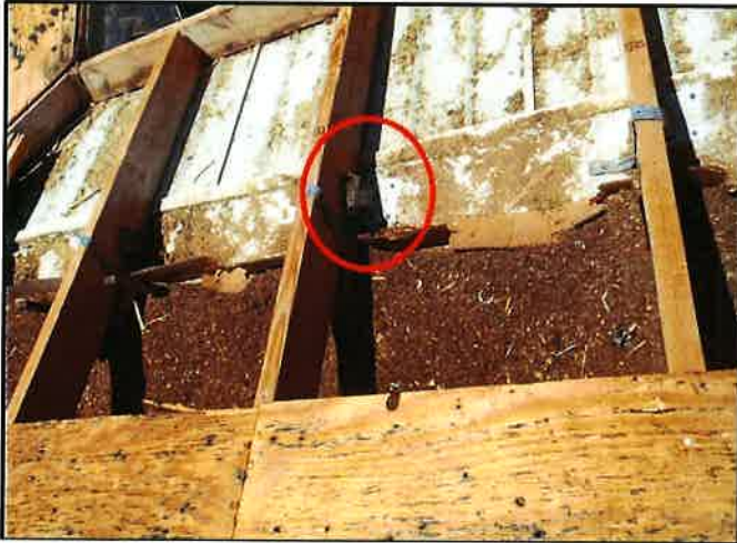
Truss to Wall Reinforcement
