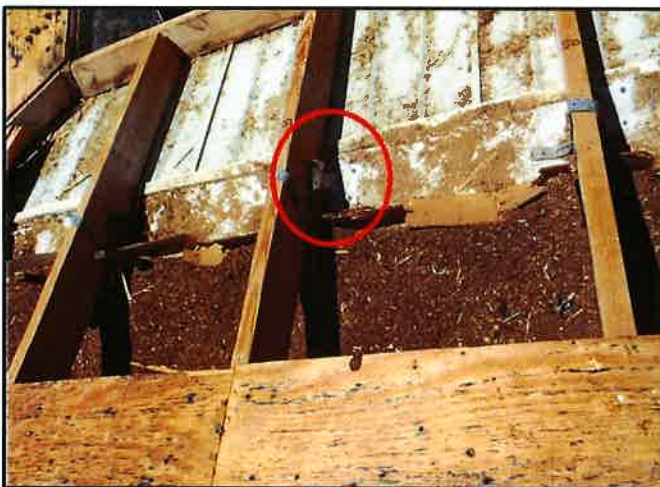
Truss to Wall Reinforcement
