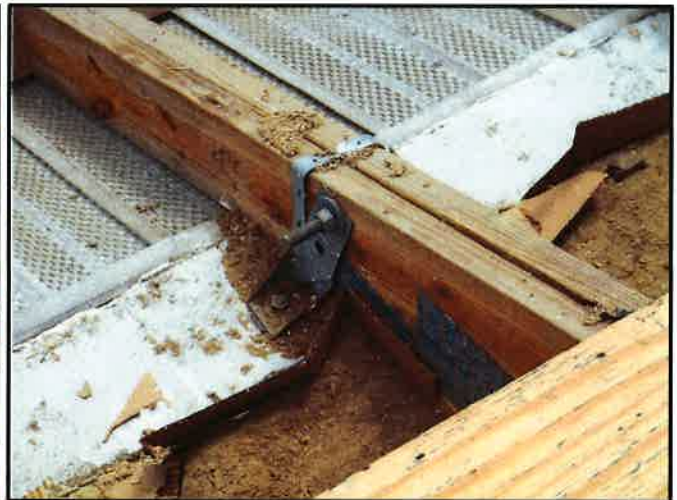
Double Truss Connection
