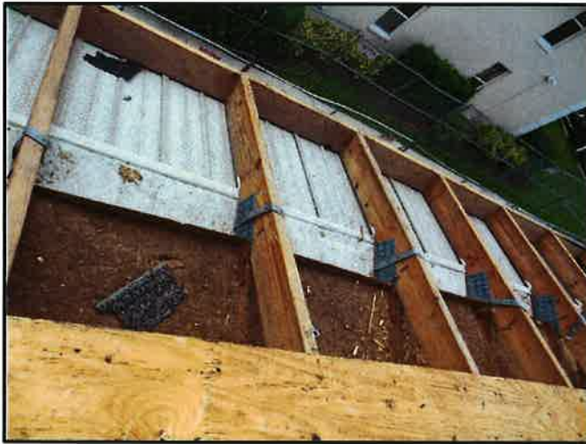
Truss Strapping
