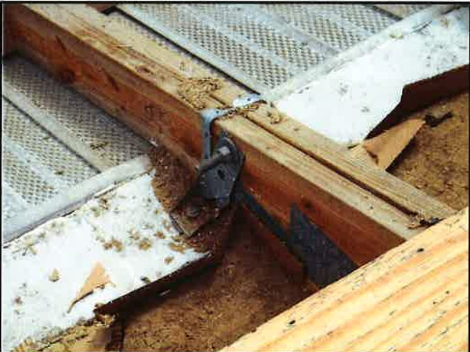
Double Truss Connection
