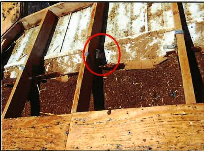
Truss to Wall Reinforcement
