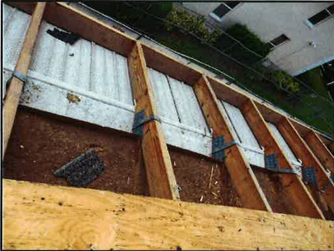
Truss Strapping
