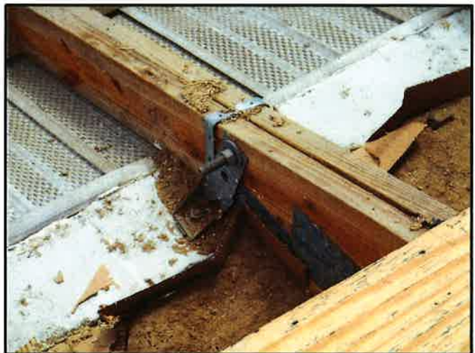
Double Truss Connection
