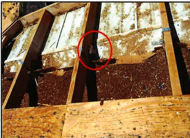
Truss to Wall Reinforcement
