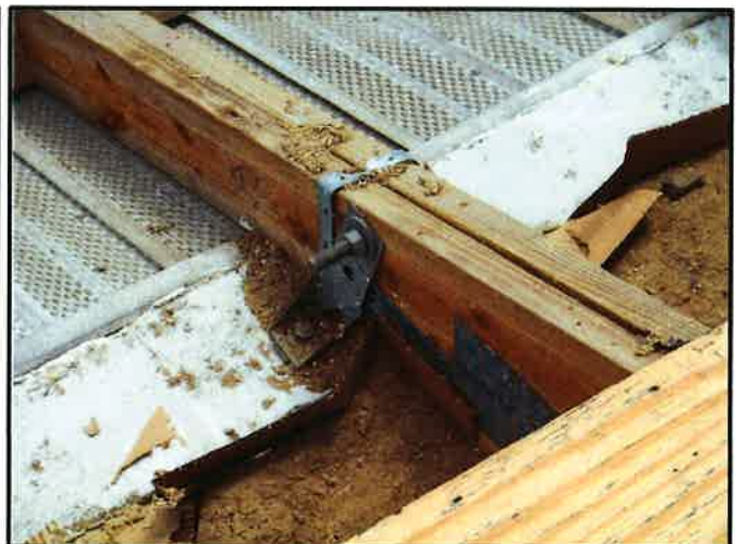
Double Truss Connection
