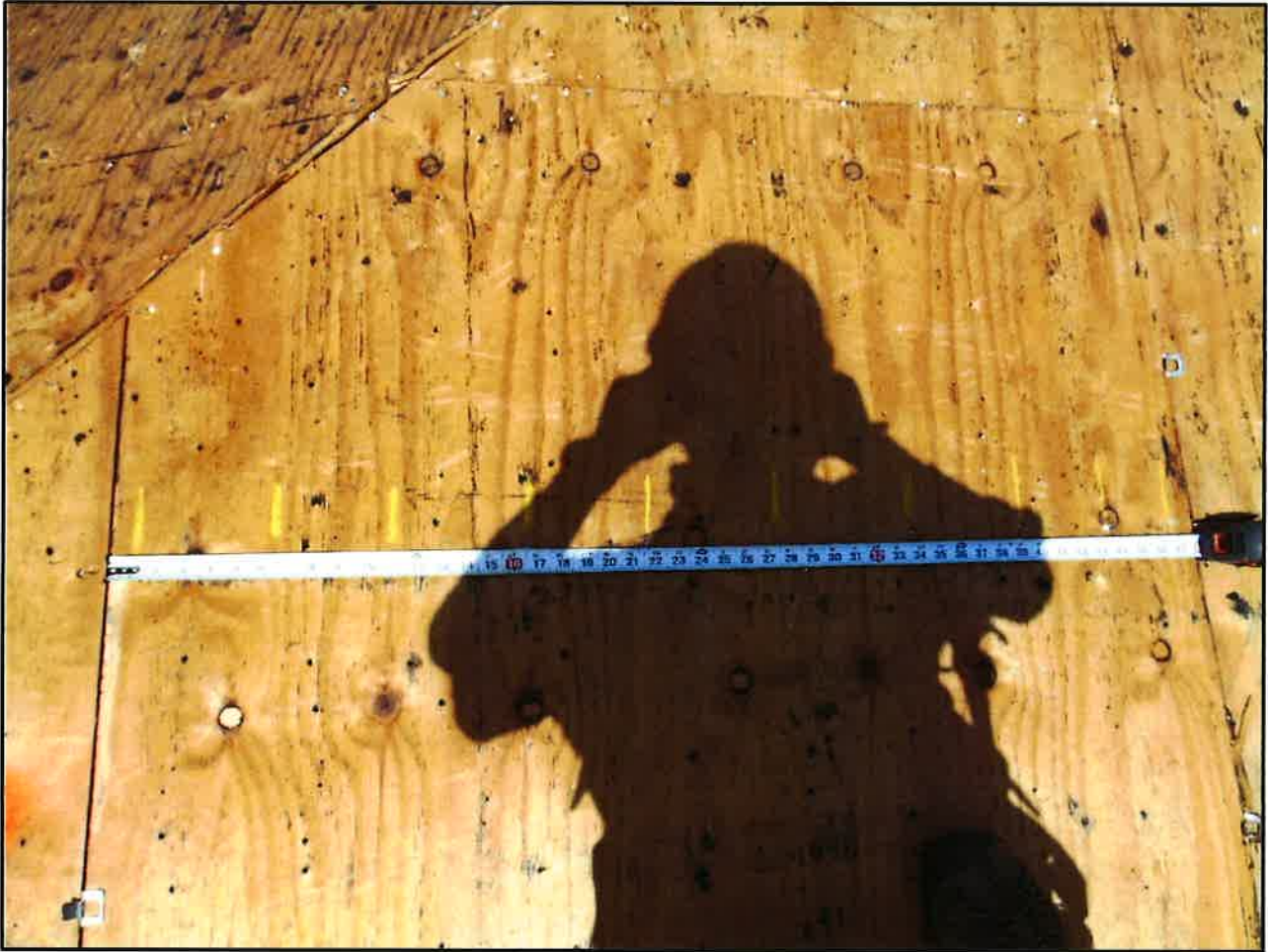
Plywood Nailing
