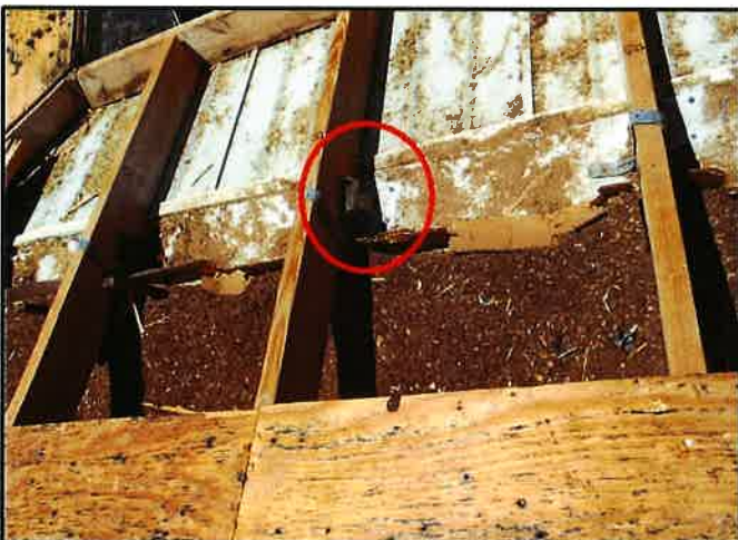
Truss to Wall Reinforcement
