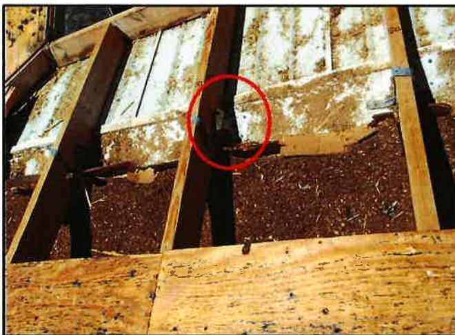
Truss to Wall Reinforcement
