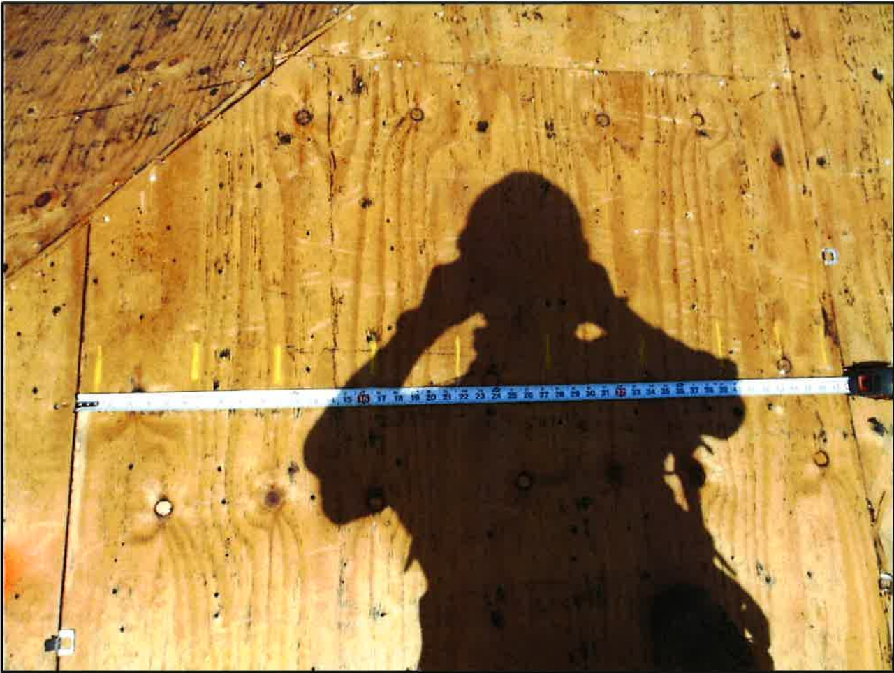
Plywood Nailing
