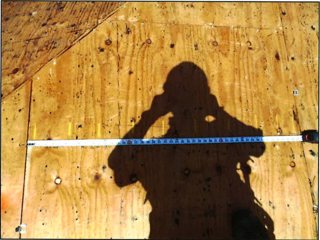
Plywood Nailing
