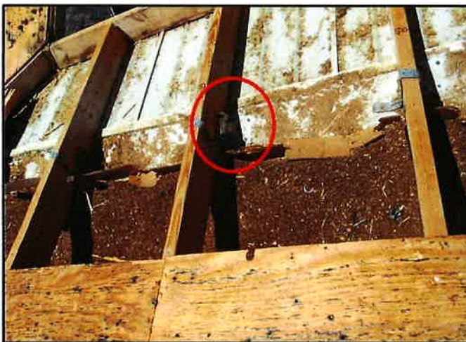
Truss to Wall Reinforcement
