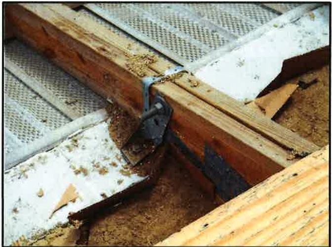
Double Truss Connection
