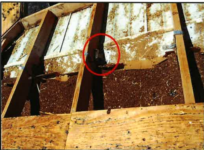
Truss to Wall Reinforcement
