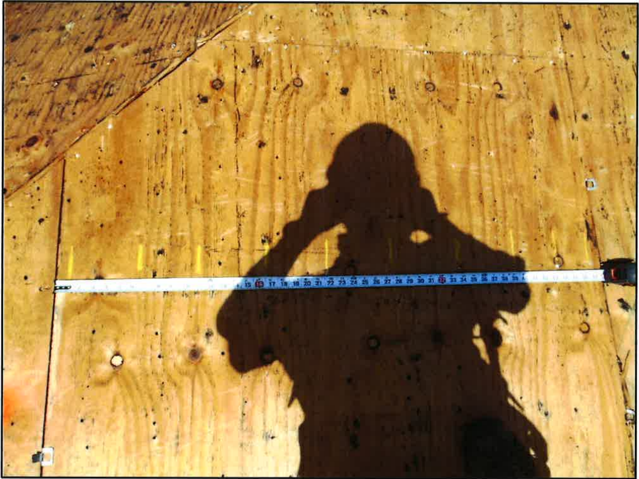
Plywood Nailing
