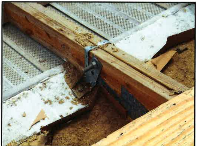
Double Truss Connection
