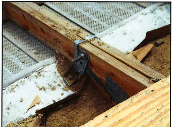
Double Truss Connection
