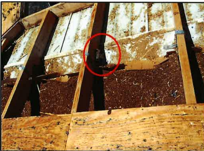
Truss to Wall Reinforcement
