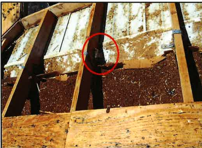
Truss to Wall Reinforcement
