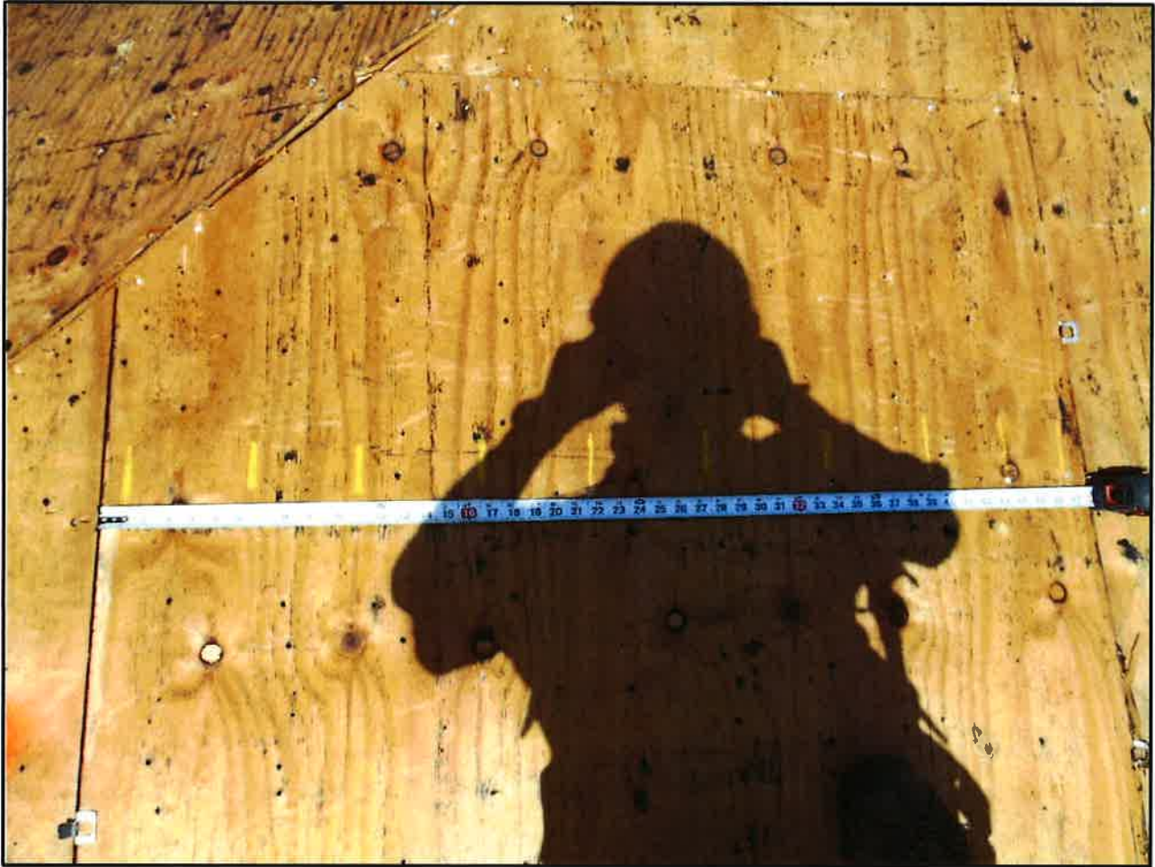
Plywood Nailing
