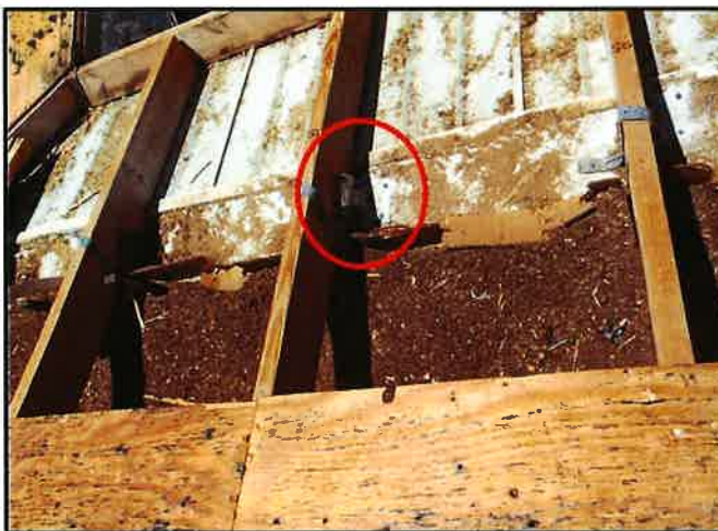
Truss to Wall Reinforcement
