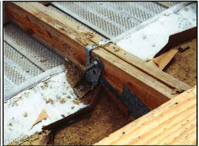
Double Truss Connection
