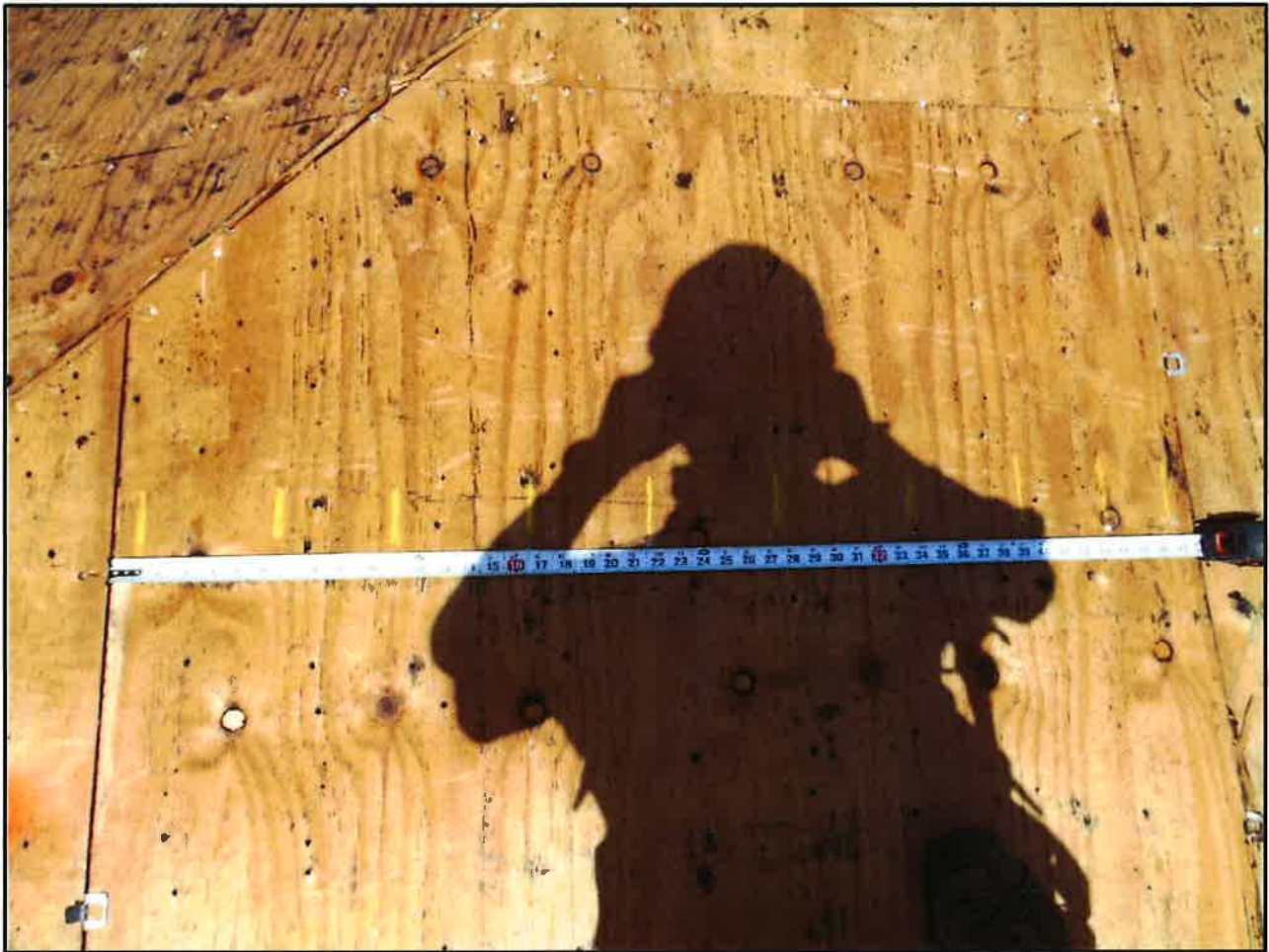
Plywood Nailing
